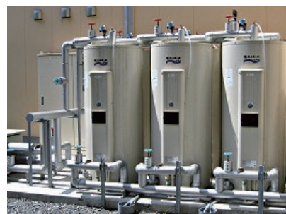
Parallel-connection water heating system for industrial uses
