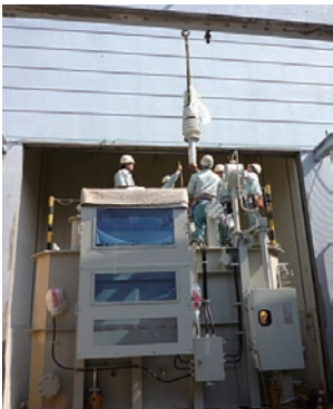
Installation of transformer
