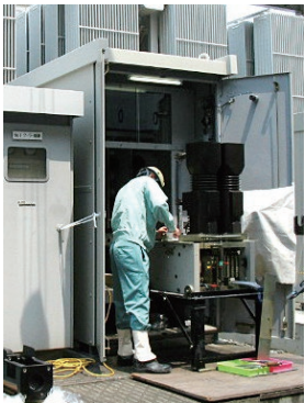
Repair of switchgear
