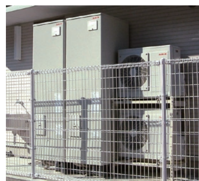
Heat pump water heaters with two connected tanks
