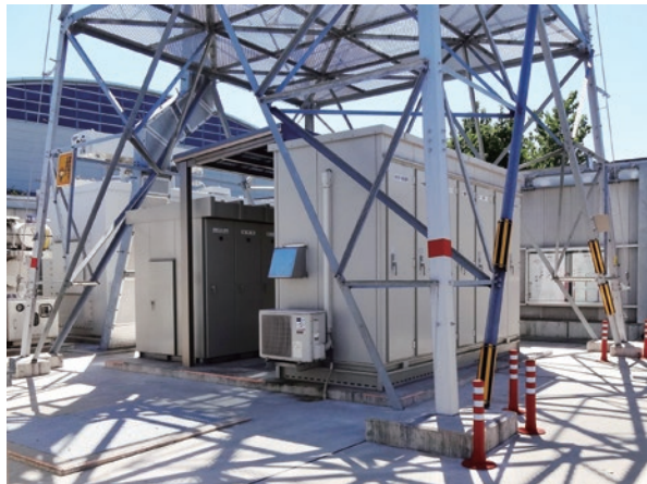
A substation within the premise of a transmission tower
