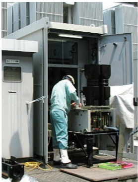
Repair of switchgear
