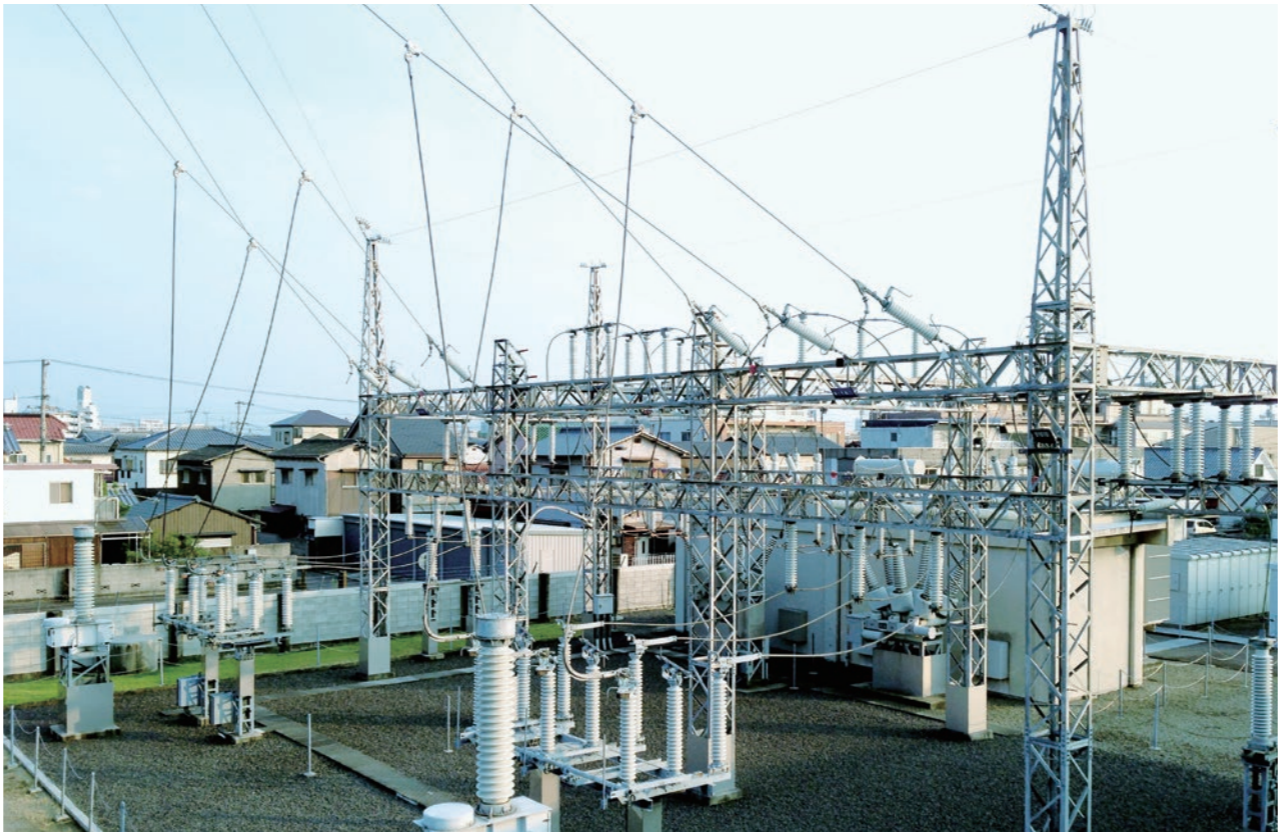
66kV distribution substation (Installed at Shikoku Electric Power Company , Incorporated )
