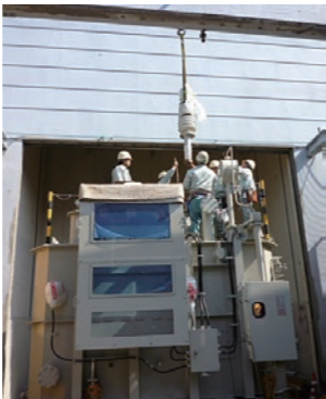
Installation of transformer
