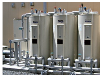
Parallel-connection water heating system for industrial uses
