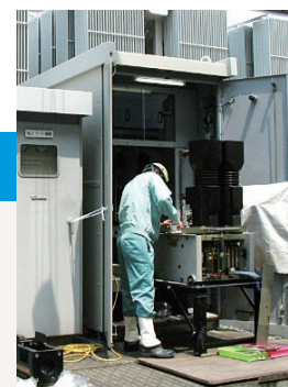
Repairing a switchgear
