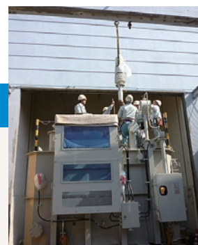
Installing a transformer
