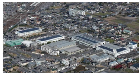
Solar panels (shown in blue)
