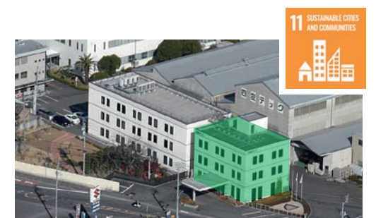
Temporary evacuation site
