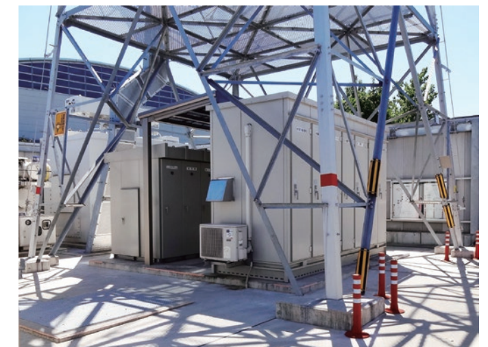
A substation on the site of a transmission tower
