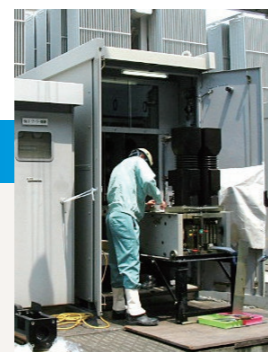
Repairing a switchgear
