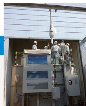
Installing a transformer
