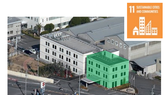
Temporary evacuation site
