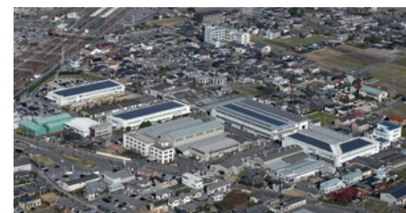
Solar panels (shown in blue)
