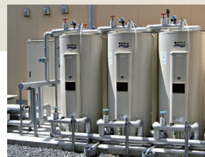
Commercial parallel hot water supply system
