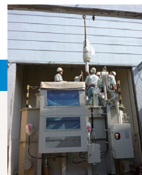
Installing a transformer
